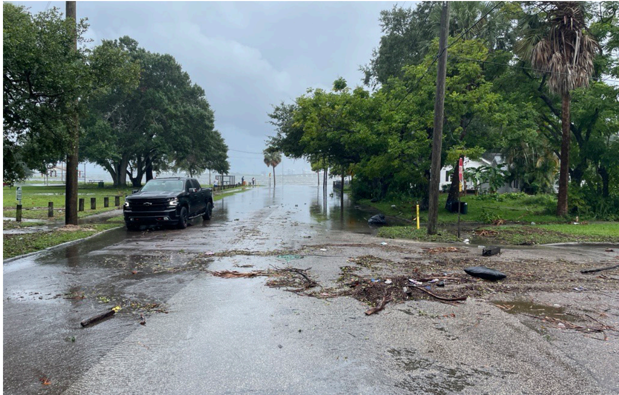
Rack line shown in post-surge condition from Hurricane Idalia, August 30, 2023 - at elevation 5.42 NAVD.
