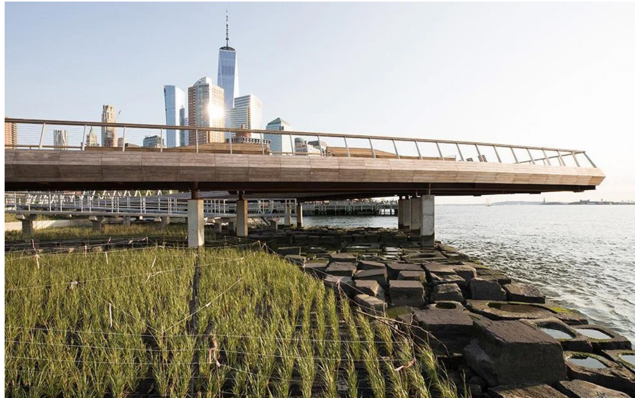
Image: Pier 26 at Hudson River Park in New York City
