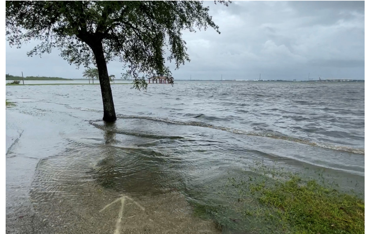
Seawall overtopping from Hurricane Idalia.
